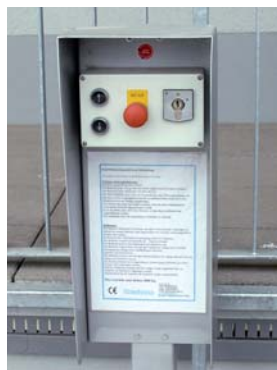
Berlin control unit with weatherproof casing and pillar
