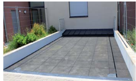
Rubber covering in stone structure (3 cm thick)
