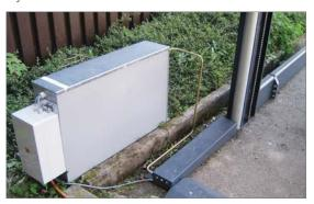
Hydraulic unit "Silencio" with tubing and wiring to the installation. The oil submerged motor "Silencio" is extremely quiet and smooth running. The motor-pump assembly is sound absorbent.
